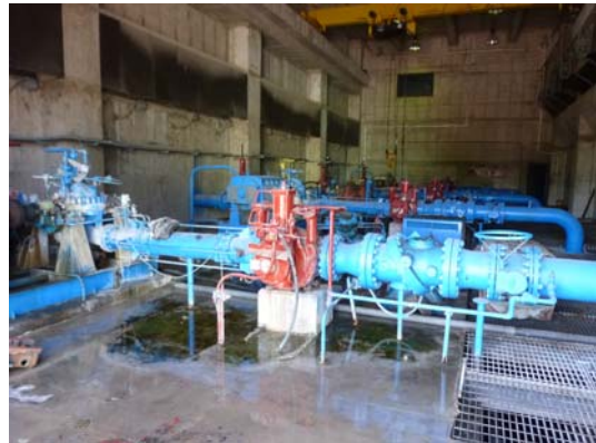
WADI-ARAB Pumping Station No. 1
