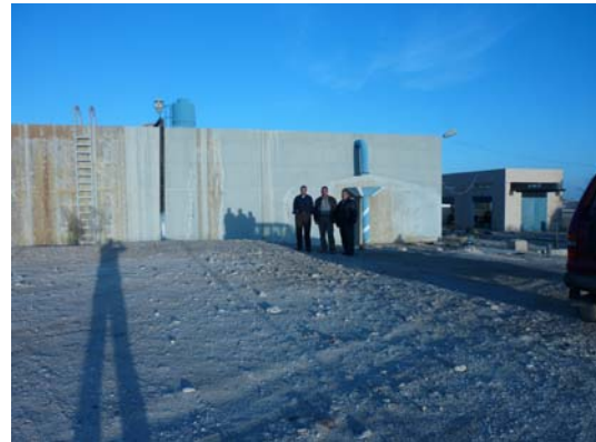
Ma'an Main Reservoir
